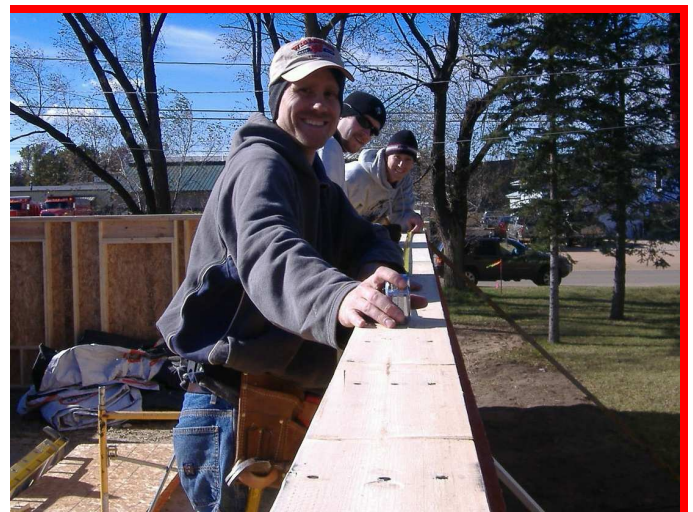
Habitat for Humanity crew preparing walls for trusses
